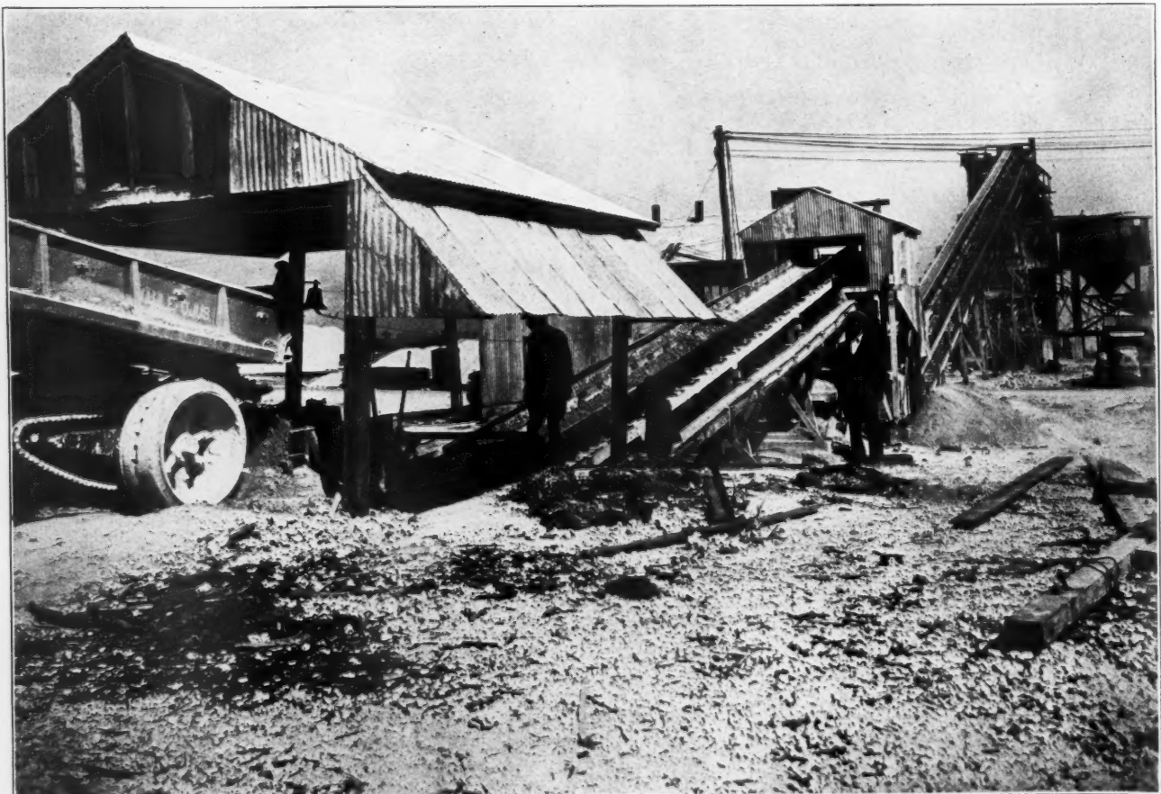
Material Being Discharged at Plant by Truck
